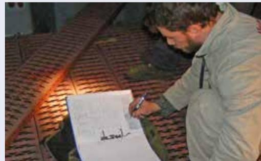
APC's MarineLine® has set the highest standards in the market with regards to heat curing and spark testing the tank surface. Heat curing enables the coating to fully cross-link so that it becomes virtually impermeable. Spark testing ensures that the cargo tank is coated properly without any voids.
