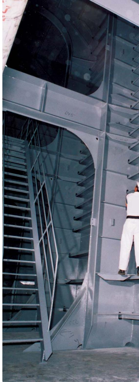
by chlorides or hydrocarbons. These tests are easily administered and verified immediately. If the steel is found to be contaminated, it will be necessary to wash the tank with a solution to remove either or both contaminants prior to blasting. Another recommended practice at this time is to check the welds, pits and steel for any other potential problems that may have been exposed during the initial blast.
