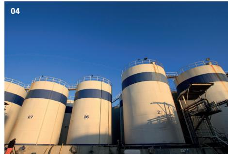
thousand aggressive chemicals including H<sub>2</sub>SO<sub>4</sub>, waste acids, 37% HCl, acetic acid, and other aggressive acids, caustic soda, alkalis, solvents, hot oils, fracking materials, brine, edible oils, and others.
