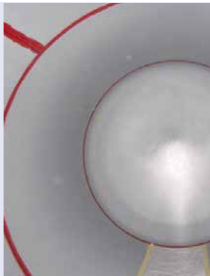
Initial application work on Solvay rail tankcars. Two coats of ChemLine®, a grey base coat followed by a red top coat.
