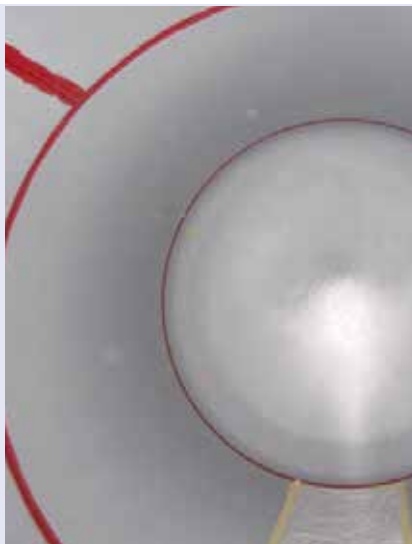
Initial application work on Solvay rail tankcars. Two coats of ChemLine®, a grey base coat followed by a red top coat.
