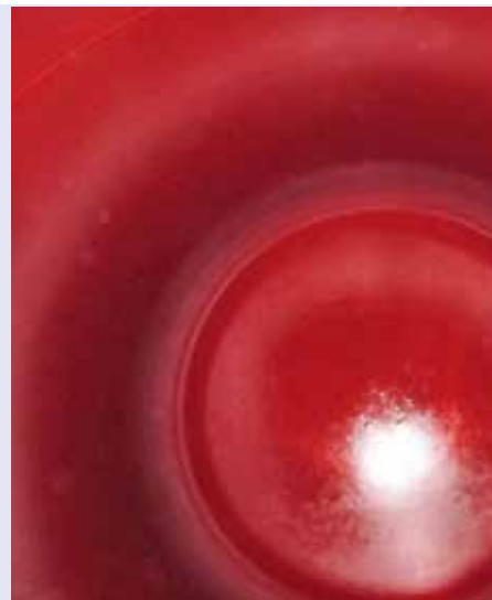
Initial application work on Solvay rail tankcars. Two coats of ChemLine®, a grey base coat followed by a red top coat.
