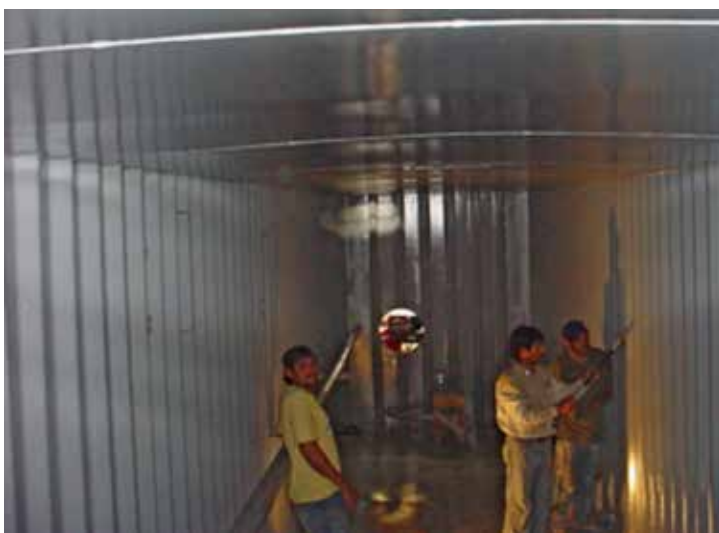
(Top) Fracking tank being readied for internal lining application of ChemLine® 784/32. (Bottom) Inspecting the ChemLine® 784/32 protective coating.
