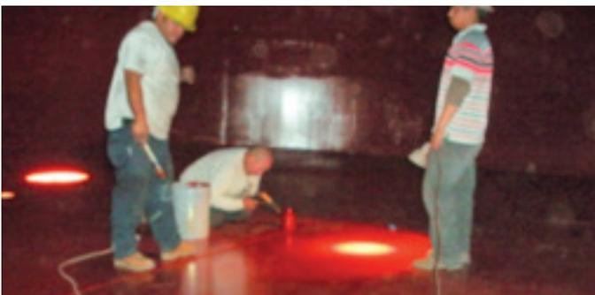
784-32 (gray) to the roof and walls and at 6-8 mils (150-200) microns wet film thickness in accordance to the specification.
