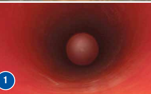
1) Interior pitted OTR tank with corrosion prior to ChemLine® application, and then coated with protective ChemLine®. 2) Manway lid showing corroded rubber lining, due to HCL exposure, and manway lid and surrounding spill area then properly protected with ChemLine® coating. 3) ChemLine® coating application.
