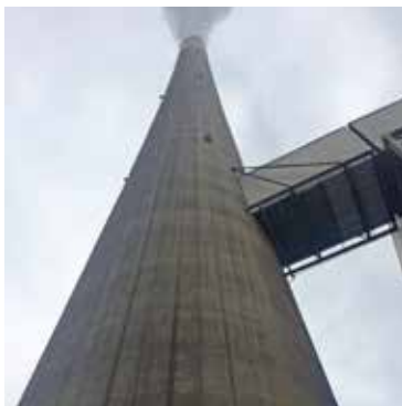
(Left) At this coal-fired power facility the 180 meter high, carbon steel stack lined with a competitor's coating severely delaminated only after 10 months of service as this photo (center) shows near the top of the stack. Normal operating temperature is around 140°F/60°C but at times it reaches up to 233°F/112°C. (Right) After blasting out the previous coating, the top section of the stack is now lined with ChemLine® and
