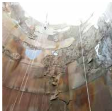
(Left) At this coal-fired power facility the 180 meter high, carbon steel stack lined with a competitor's coating severely delaminated only after 10 months of service as this photo (center) shows near the top of the stack. Normal operating temperature is around 140°F/60°C but at times it reaches up to 233°F/112°C. (Right) After blasting out the previous coating, the top section of the stack is now lined with ChemLine® and
