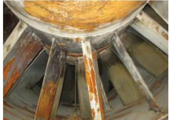
*Booster fans exhibit severe corrosion problems and need to be coated.*
