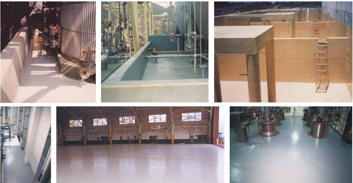
ChemLine® is used extensively to protect secondary containment areas and concrete flooring at chemical processing facilities, tank farms, and other high performance areas.
