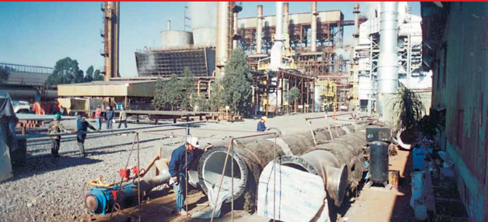
(Above) Spark testing the ChemLine® lining of the pipe before installation.
