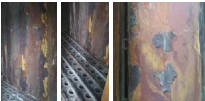
(Top) Severe corrosion inside Baghouse. (Bottom) ChemLine® coating applied.
